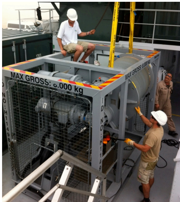
Figure 26: CTD Winch with .322 cable drum being fitted. The winch is located on the 4 th deck aft, forward of the helideck.
