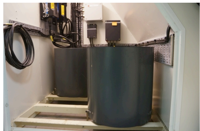
Figure 12: Gyrocompasses sitting below the MRUs.
